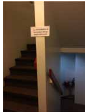
Figure 20: Staircases do not have handrails on both sides
