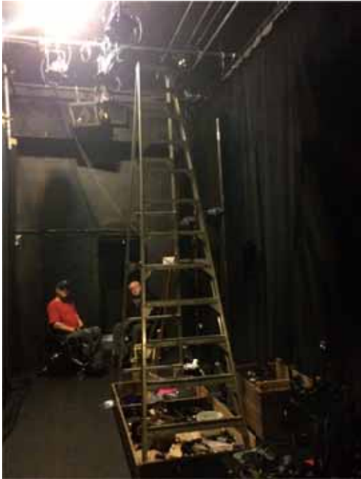
Figure 33: Ladder providing access to overhead lighting equipment
